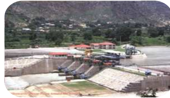
Jaypee Hydro Power Plant
